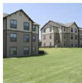
CEV Weatherford Weatherford, OK 356 Beds
